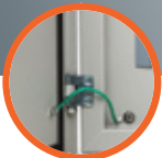
Door earthing to protect against electric shock
